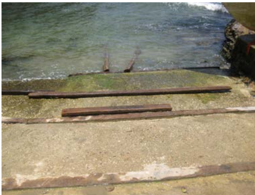
Figure 10.3 Refurbished ramp at the Blanchisseuse Fishing Facility
